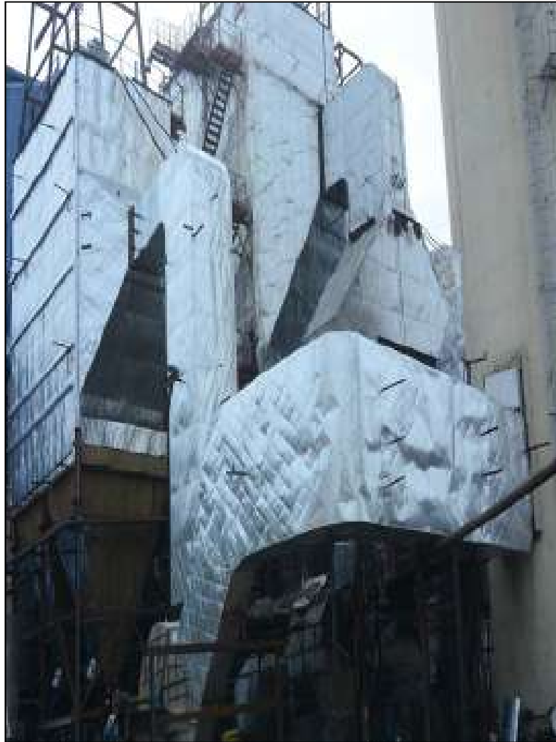
ESP for 20 & 90 TPH Boiler Capacity
