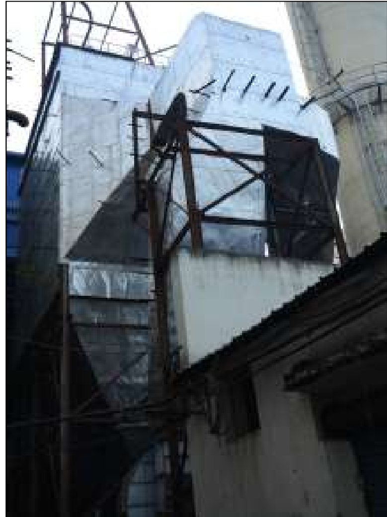
ESP for 75 TPH Boiler Capacity
